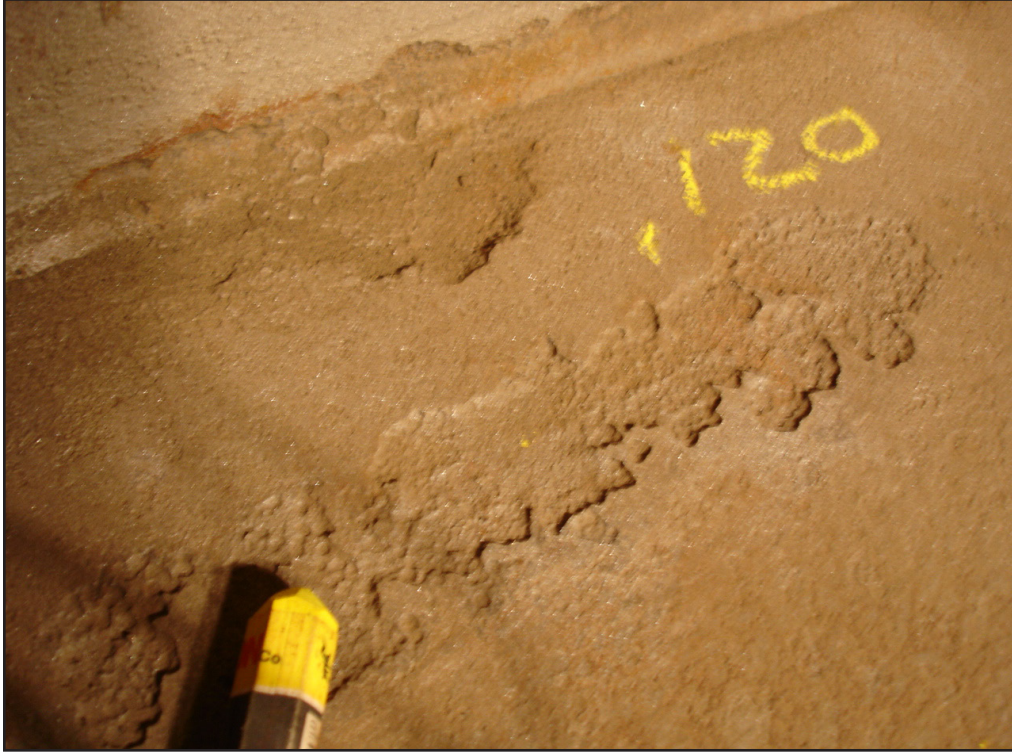
Figure 7. Pitting under UAN tank sludge.
