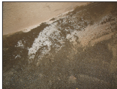
Figure 6. UAN tank sludge.
